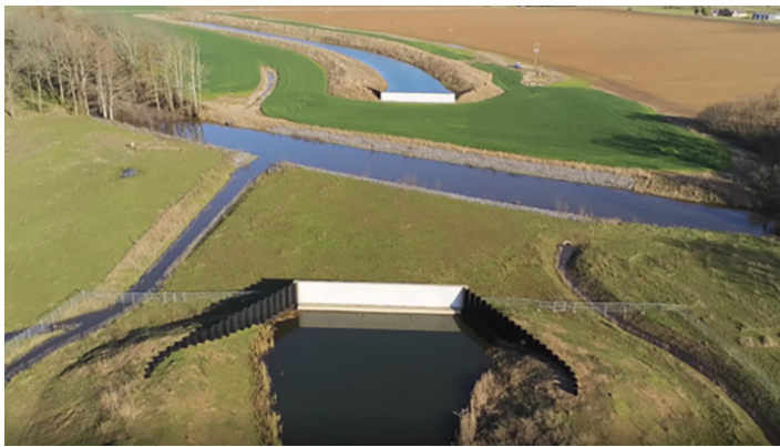
An inverted siphon under Scott Bayou.
