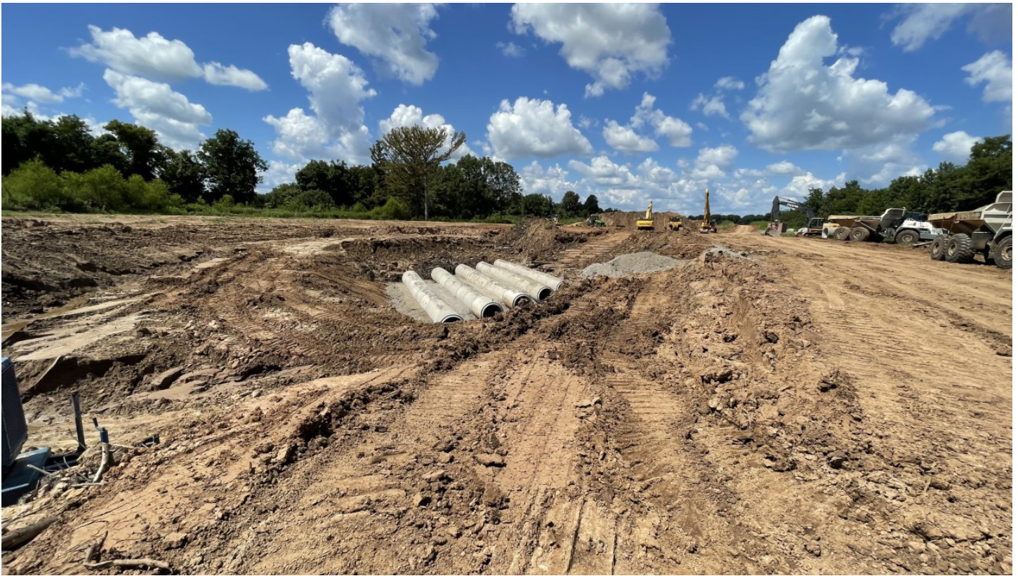
The Dry Bayou siphon, under construction.
