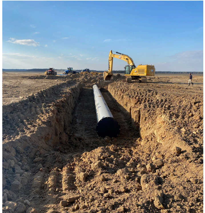
The installation of a pipe.
