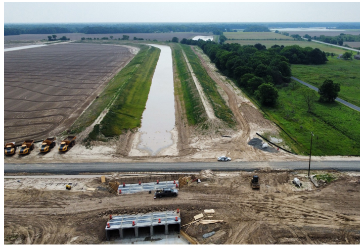
A county road crossing under construction.
