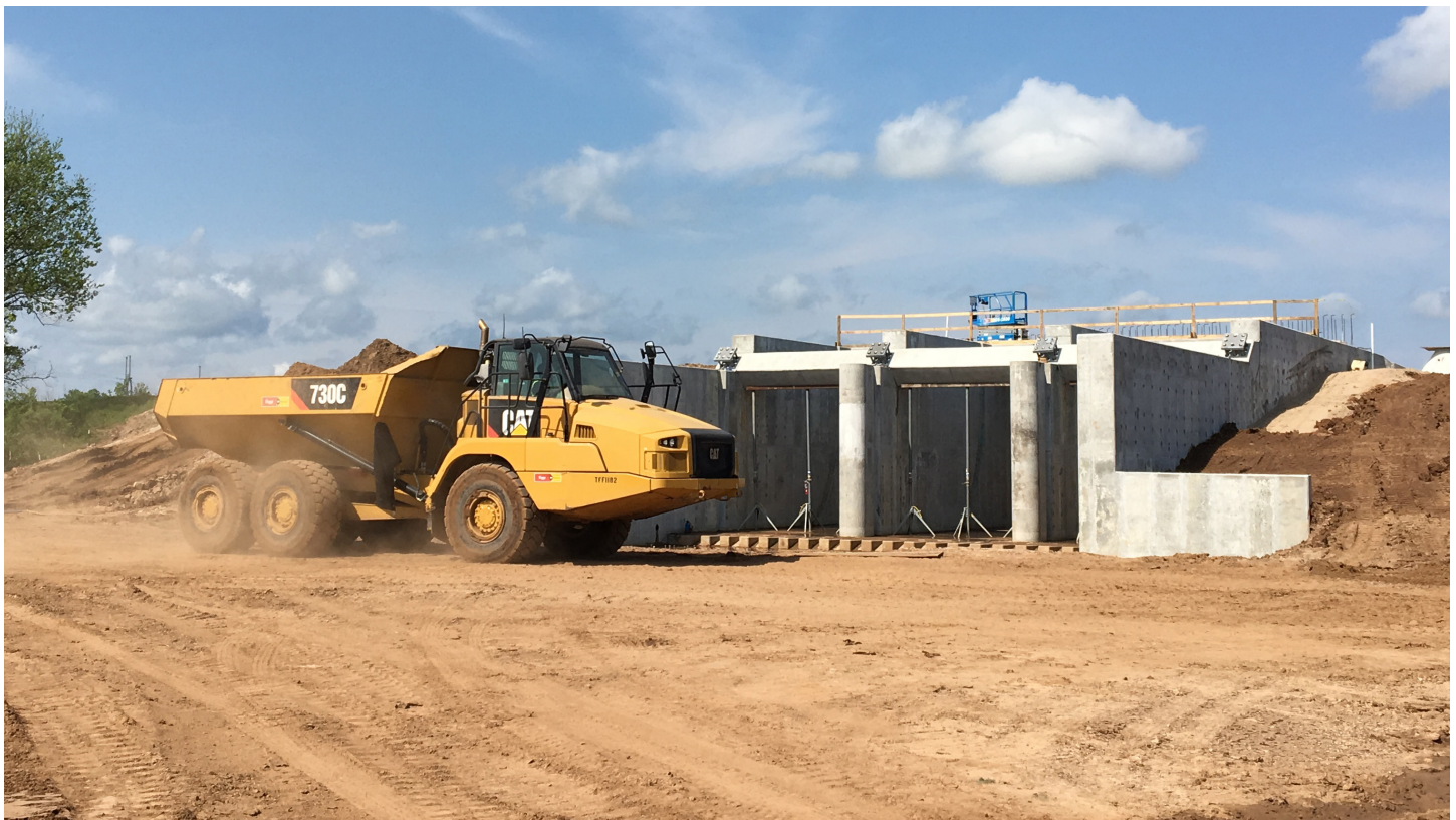
The construction of regulating reservoir gates.
