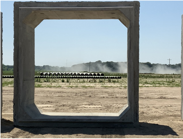
Steel pipe for landowner water offtakes and siphons (background) and concrete box culverts for road crossings (foreground) in storage.
